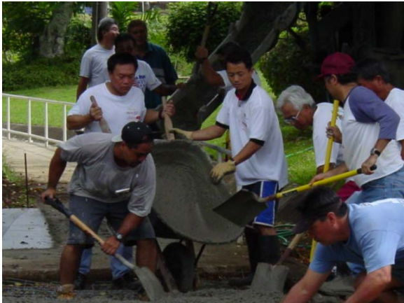
Kapunahala Elementary School—Sidewalk repair
